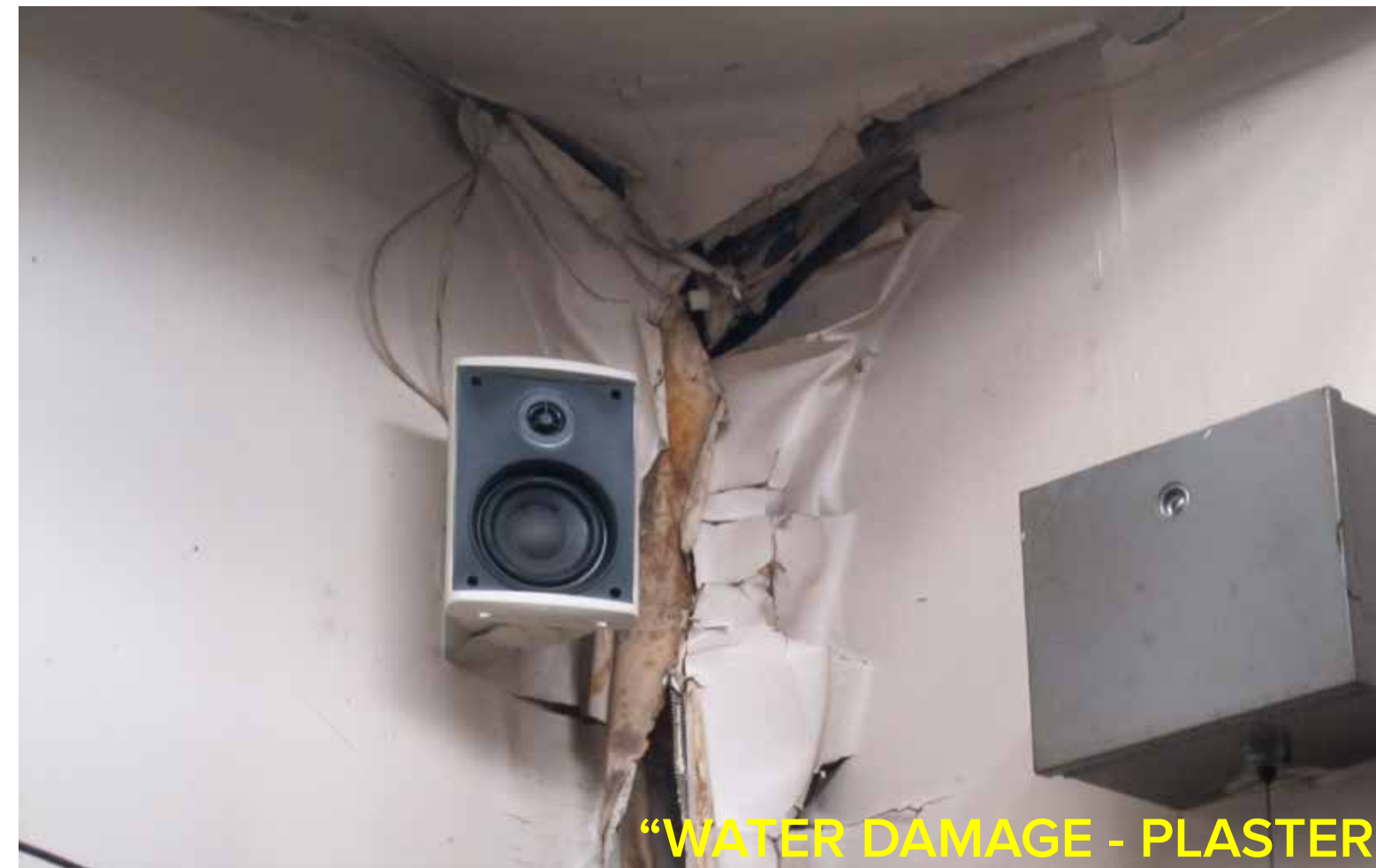
“WATER DAMAGE - PLASTER”
