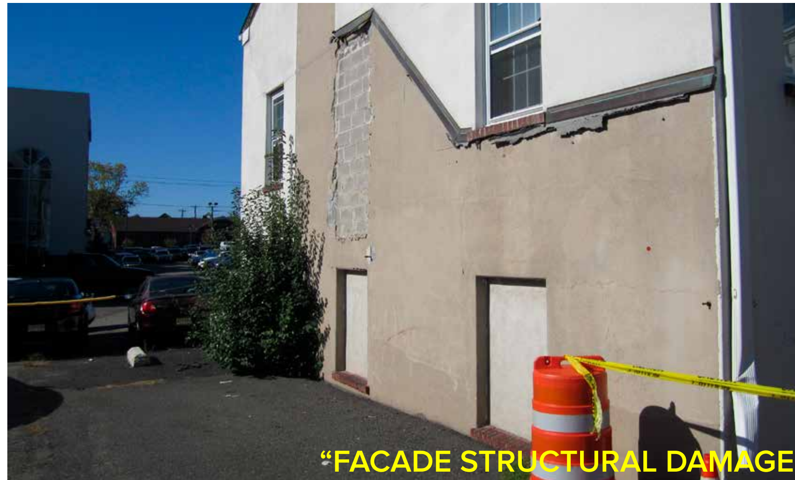
"WATER DAMAGE - STUCCO - CAN SEE DAYLIGHT"
